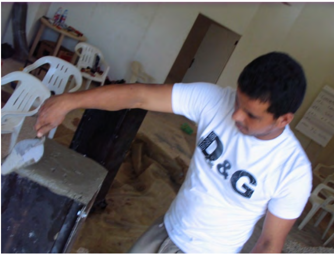
Trowelling cement in the mould.
