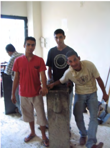
Finished concrete filter revealed!
