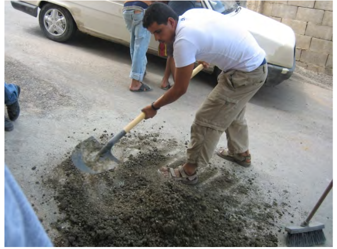
Mixing materials for cement.
