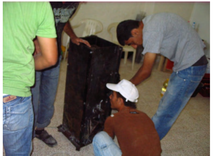
Preparing the mould for the cement pour.
