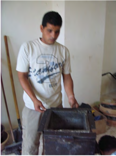
Stripping the mould from the cured concrete filter.
