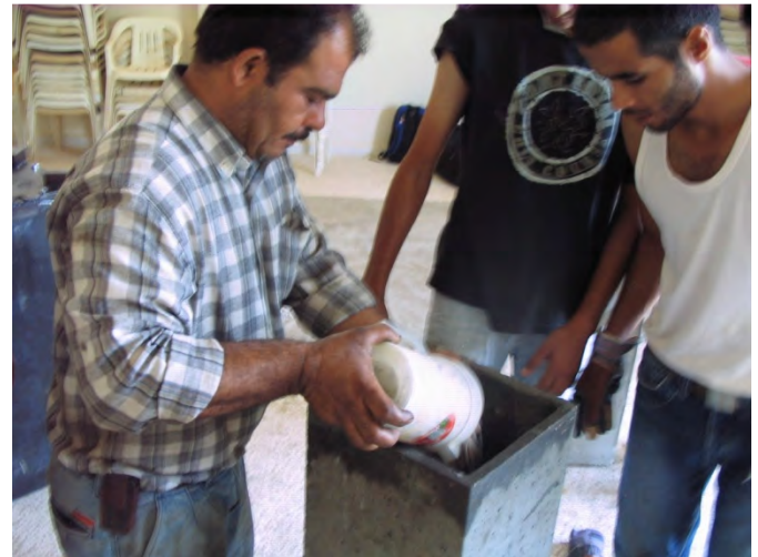
Pouring the sifted and sorted filter materials by layers into the concrete filter.
