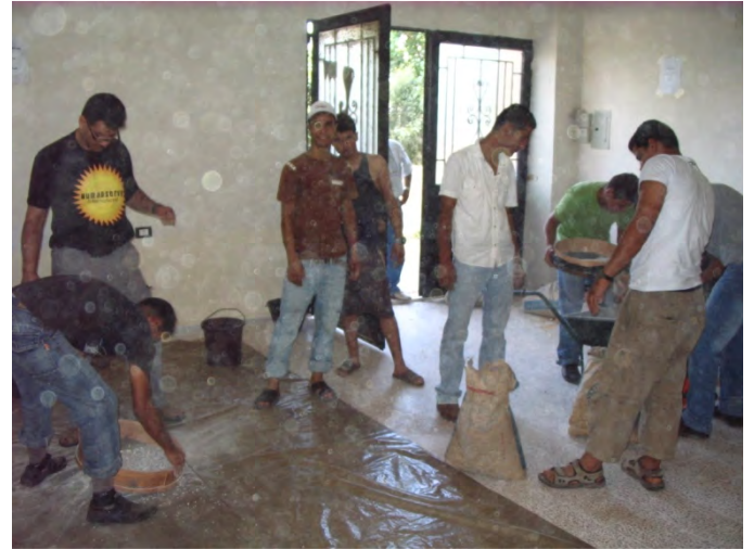
Sifting filtering materials (fine sand to large gravel)
