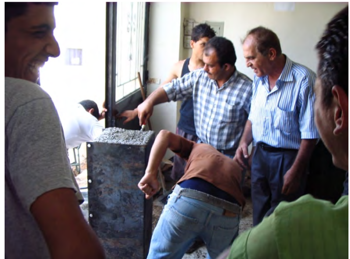
Trowelling cement in the mould.
