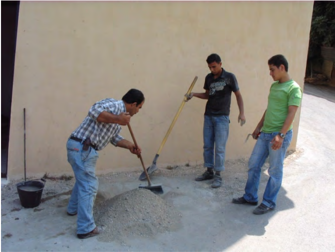
Mixing materials for cement.
